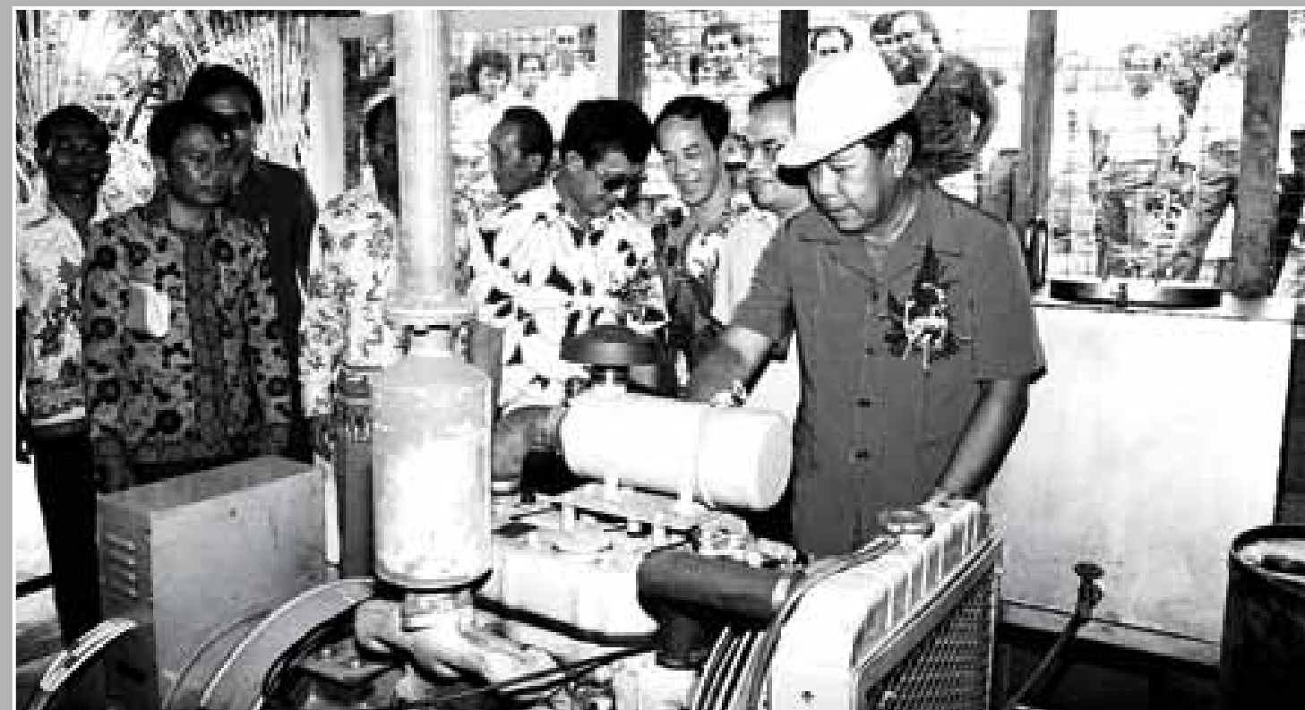
YB Dato Sri Edward Jeli officiated at the commencement of supply of electricity at Kampung Pisa, 1985.
