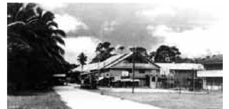
Wooden shophouses and Qi Zhi School in Long Lama Town, 1970s
