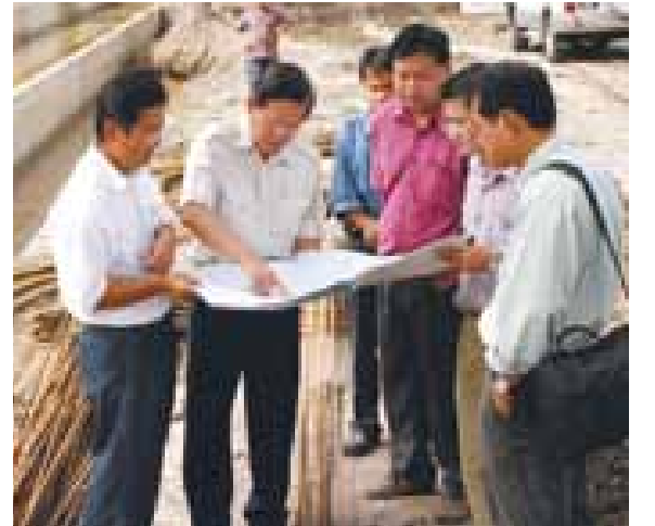
Inspecting and making sure the infrastructure projects comply to standards and requirements.
