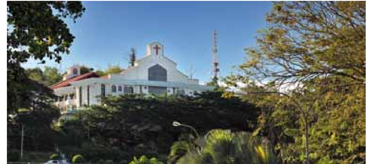
The largest church building owned by Borneo Evangelical Church (SIB) on top of Canada Hill.
